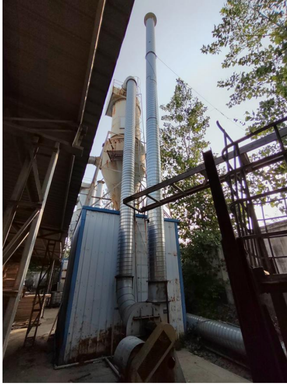
地板砂光、台锯粉尘-3#除尘器-DA004
