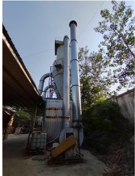
开槽粉尘-2#除尘器-DA003
